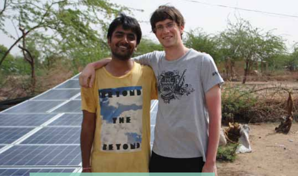
Berkeley Engineers Yashraj Khaitan and Jacob Dickinson , pictured here beside Gram Power's first microgrid solar array outside Rajasthan, India.
